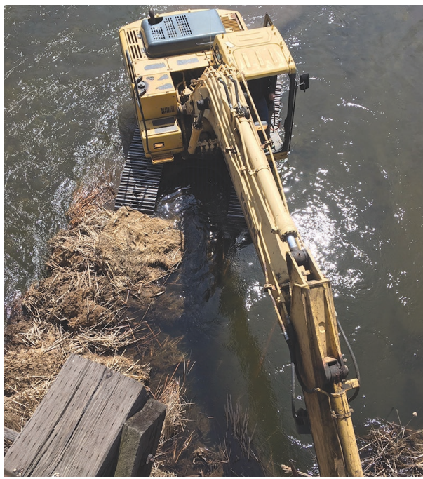
In response to a request from the Minnesota DNR, the Band contracted with Chad Milton to remove vegetation that had dammed the Rum River at the Sioux Line Trail trestle in Onamia. The dam was creating a safety hazard and causing flooded basements.
