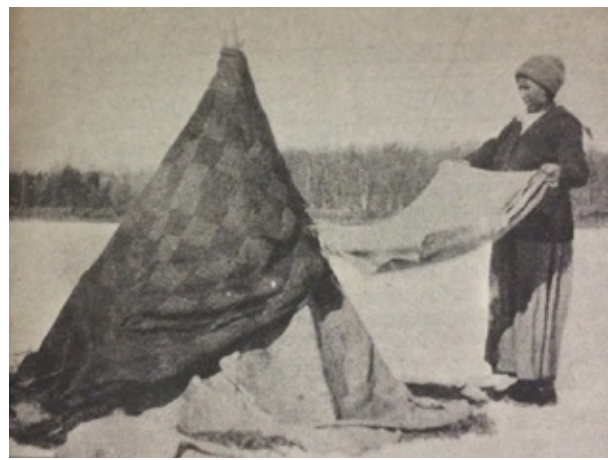
This photo from 1911 shows a traditional spearing house made of saplings and covered with blankets.
