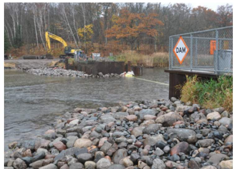
The Buck Moore Dam was removed in late October to lower the lake level and bring back the lake's wild rice beds.
