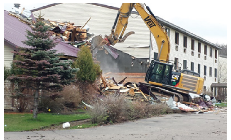
Eddy's began demolition on May 13.
